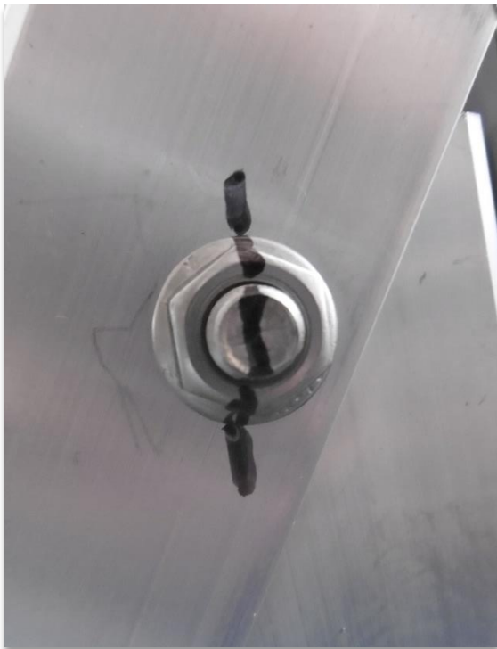
1. Mark of inspection bolt
